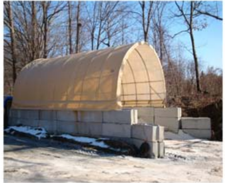
NEW SALT SHED
