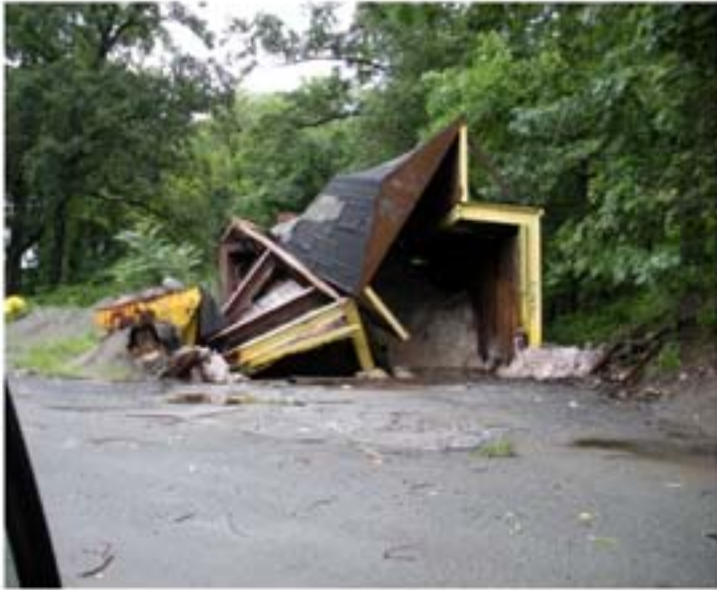
OLD SALT SHED
